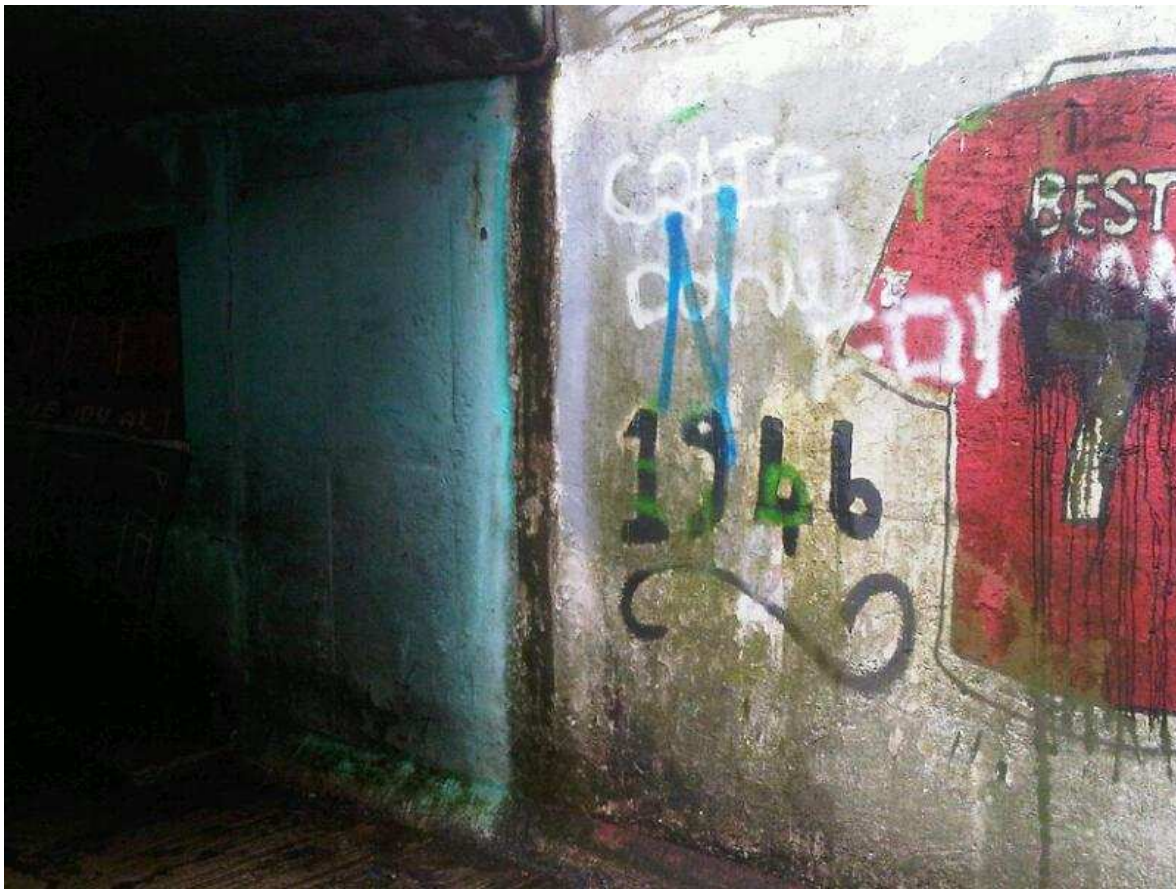
Further photos of underpass sides
